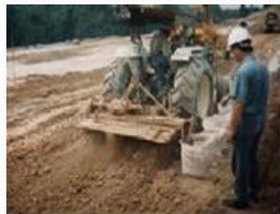
Mixing by Rotovator
